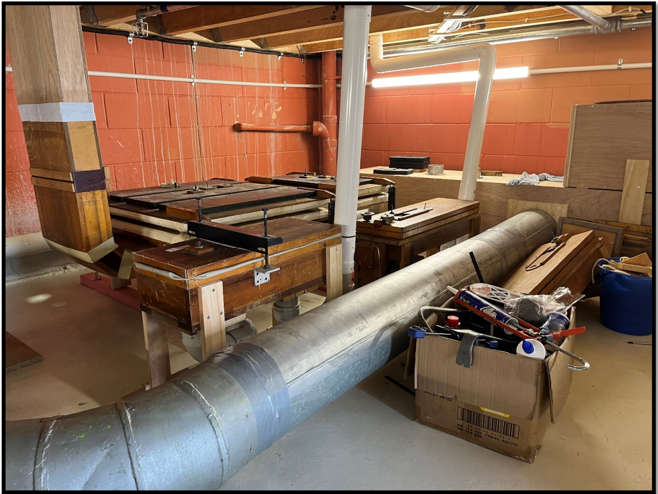
ABOVE: Another view of the Sub Chamber with Tremulants and Wind Regulators which will all feed wind up to the pipe chests in the chambers on the floor above. (Neil Warrington)
