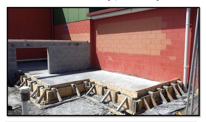
The Sub-Chamber which will house the wind regulators and tremulants with a floor being built above for the wind chests and pipes.
